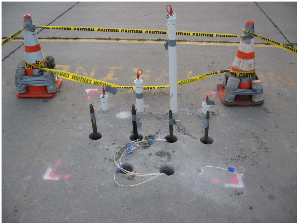
Photograph 14: PDS well, micro-purge probe, and macro-purge probe installations on slab.
