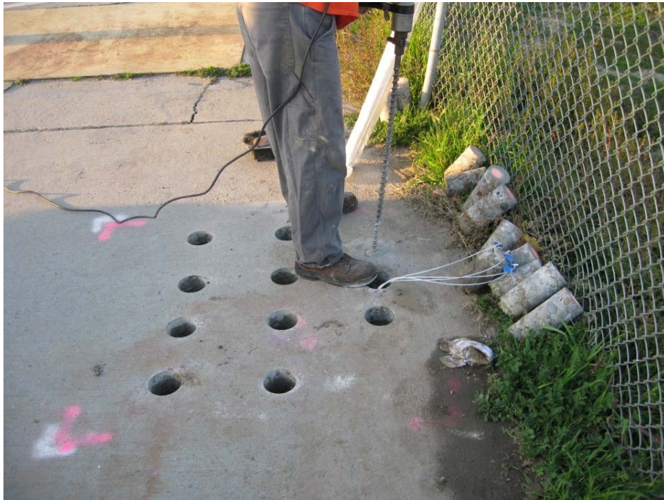
Photograph 2: Concrete core holes at location ST-2
