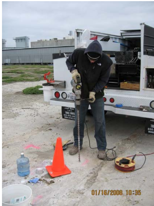
Photograph 5: Drilling hole in slab for sub-slab soil gas probe
