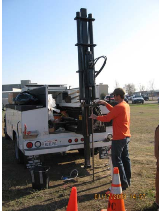
Photograph 3: Installation of macro-purge soil gas probes with H&P Stratoprobe rig.
