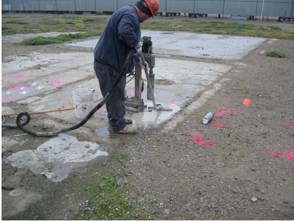
Photograph 1: Concrete coring at Building 173 slab.
