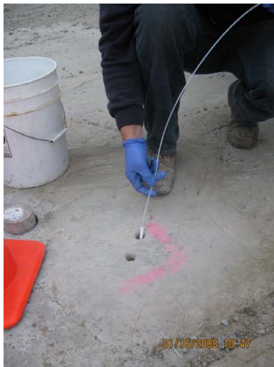
Photograph 6: Installation of sub-slab soil gas probe.
