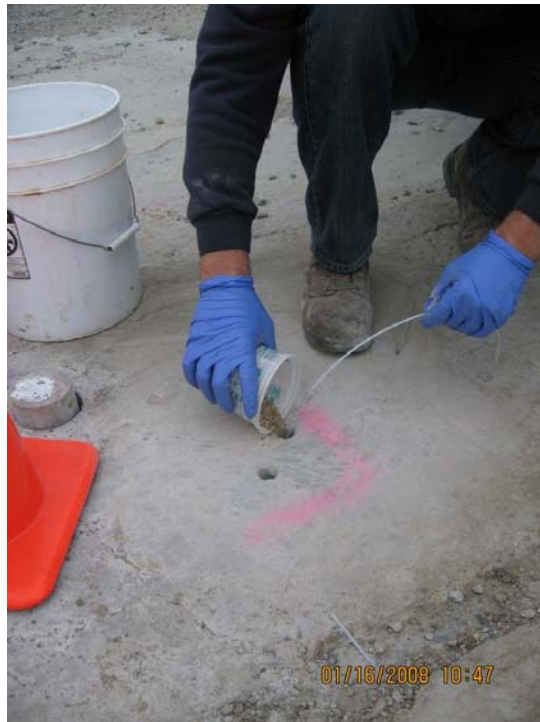
Photograph 7: Pouring sandpack for sub slab soil gas probe.
