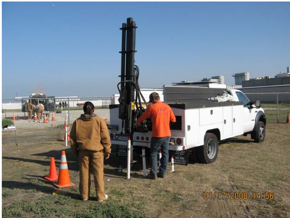
Photograph 4: Installation of PDS wells.
